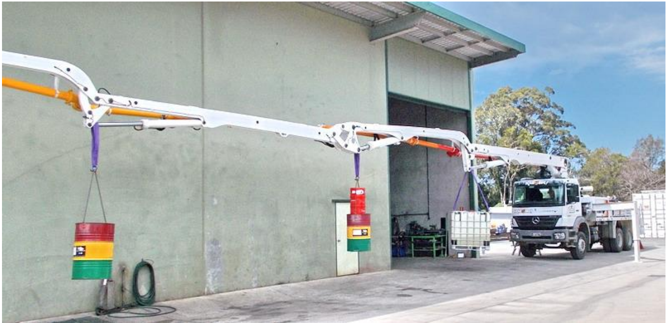
Fig 3. Weight of the load test is 25 % overload in accordance to AS1418.15
