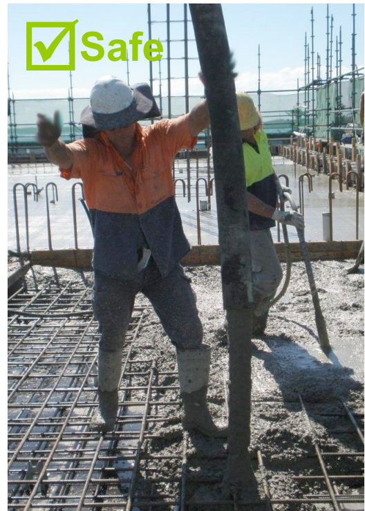
Figure 4 – Line hand guiding hose and signalling to pump operator.
