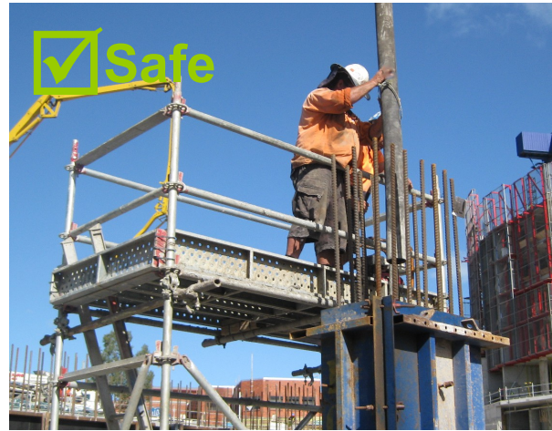
Figure 6 – Pouring concrete into column form. Good access provided
