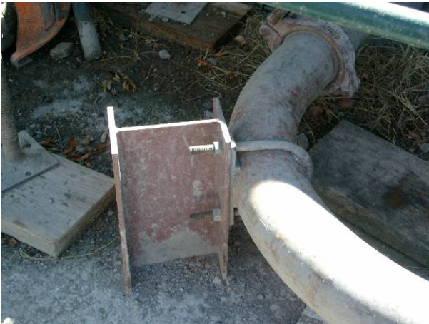
Figure 3. One method of anchoring pipe.
